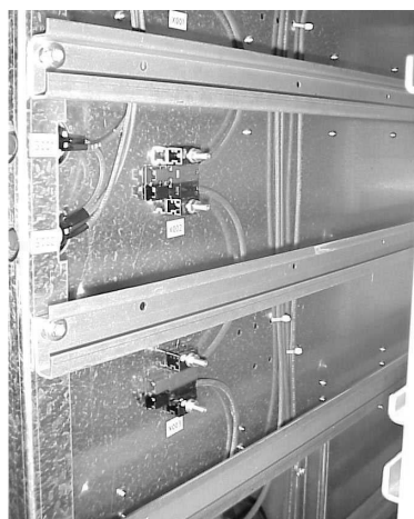
Insert battery drawers in Silcon DP300E
